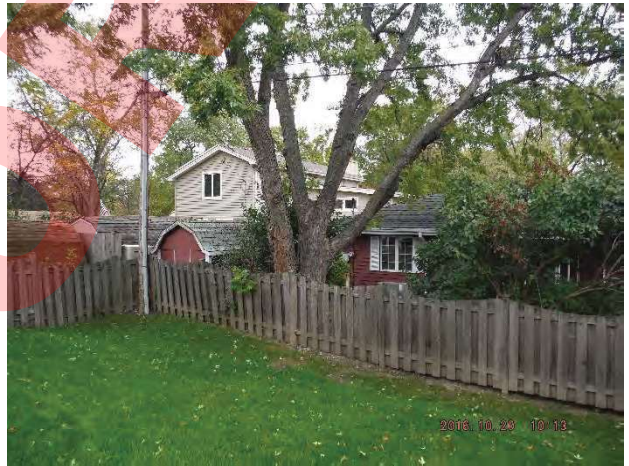
#4: Fences R&R-E; Overhead and underground utilities nearby (935 Summit's Backyard)
