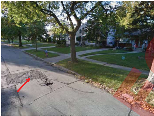
#3: MH 7-017 on Monroe St. nearby existing lateral service connection – Looking Northwest
