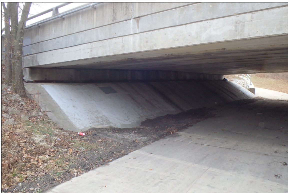
Photograph 20: View of the East Slope Wall and the Abutment, Looking Southeast.
