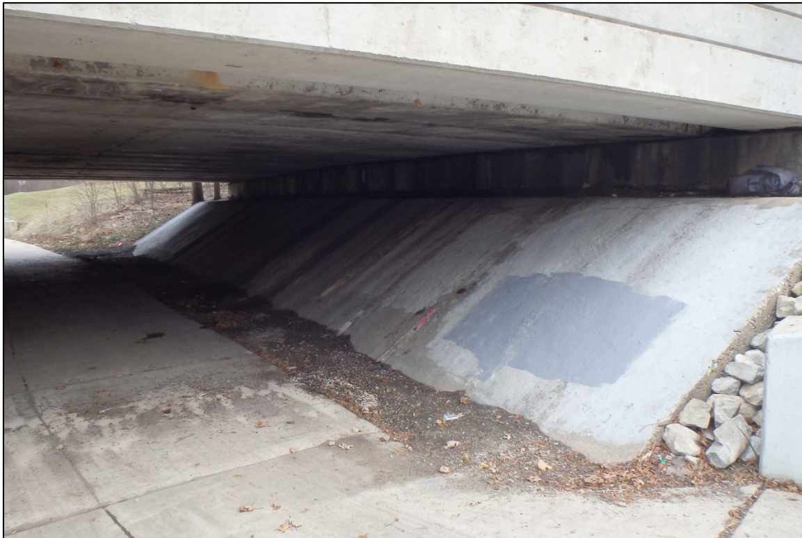
Photograph 19: View of the East Slope Wall and the Abutment, Looking Northeast.
