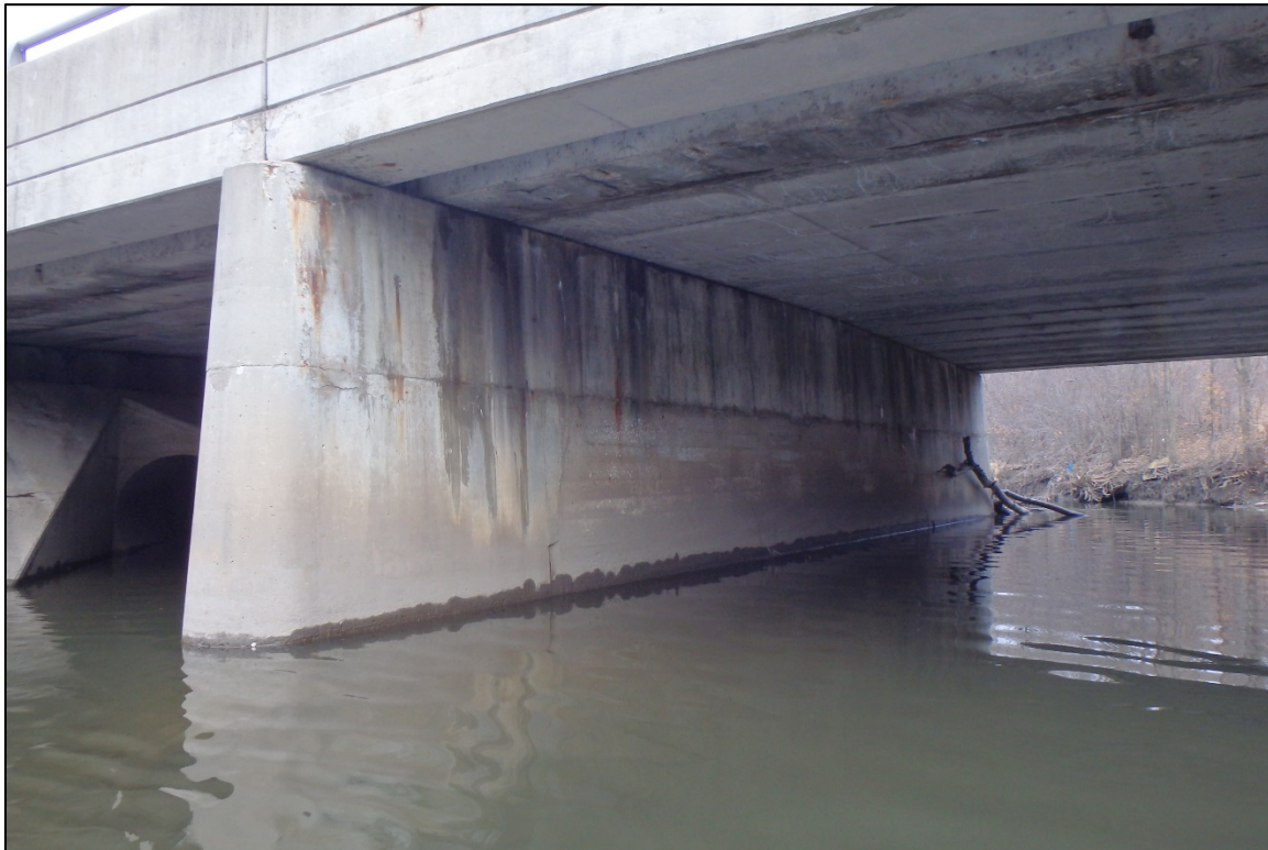
Photograph 9: View of the West Pier, Looking Northwest.
