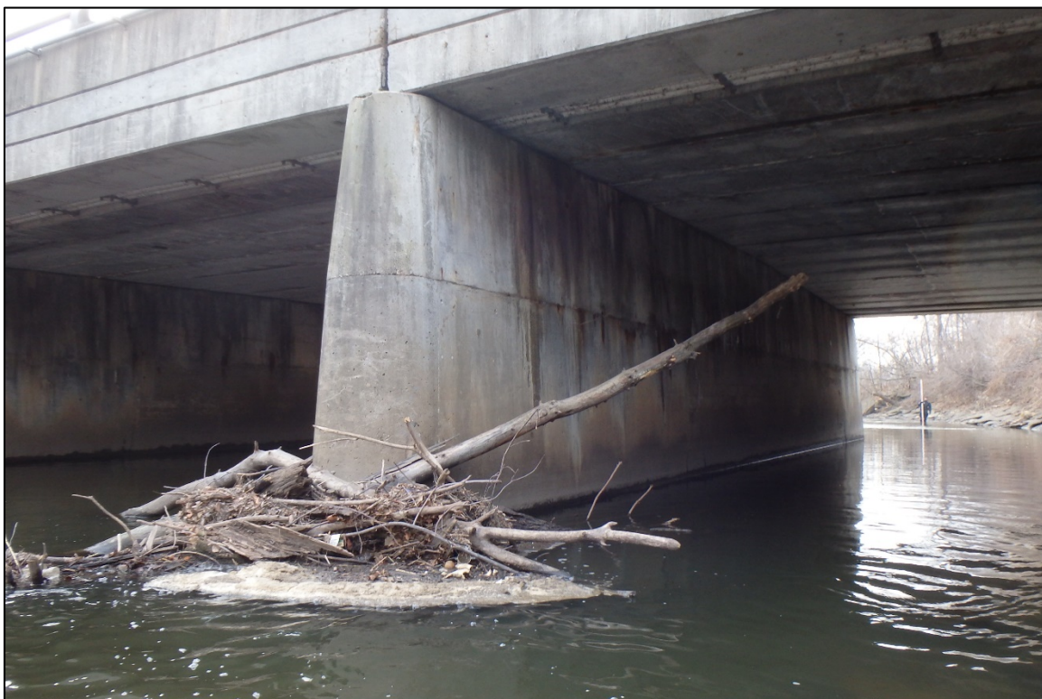
Photograph 10: View of the West Pier, Looking Southeast.
