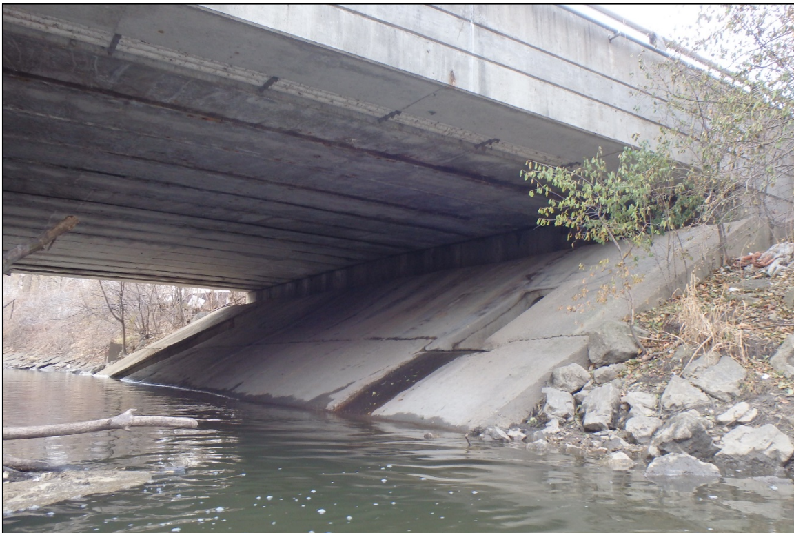
Photograph 8: View of the West Slope Wall and the Abutment, Looking Southwest.
