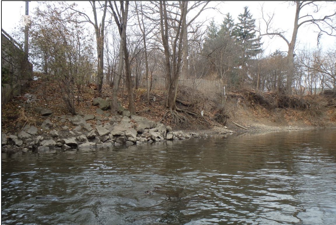
Photograph 3: View of the West Shoreline Upstream of the Bridge, Looking West.
