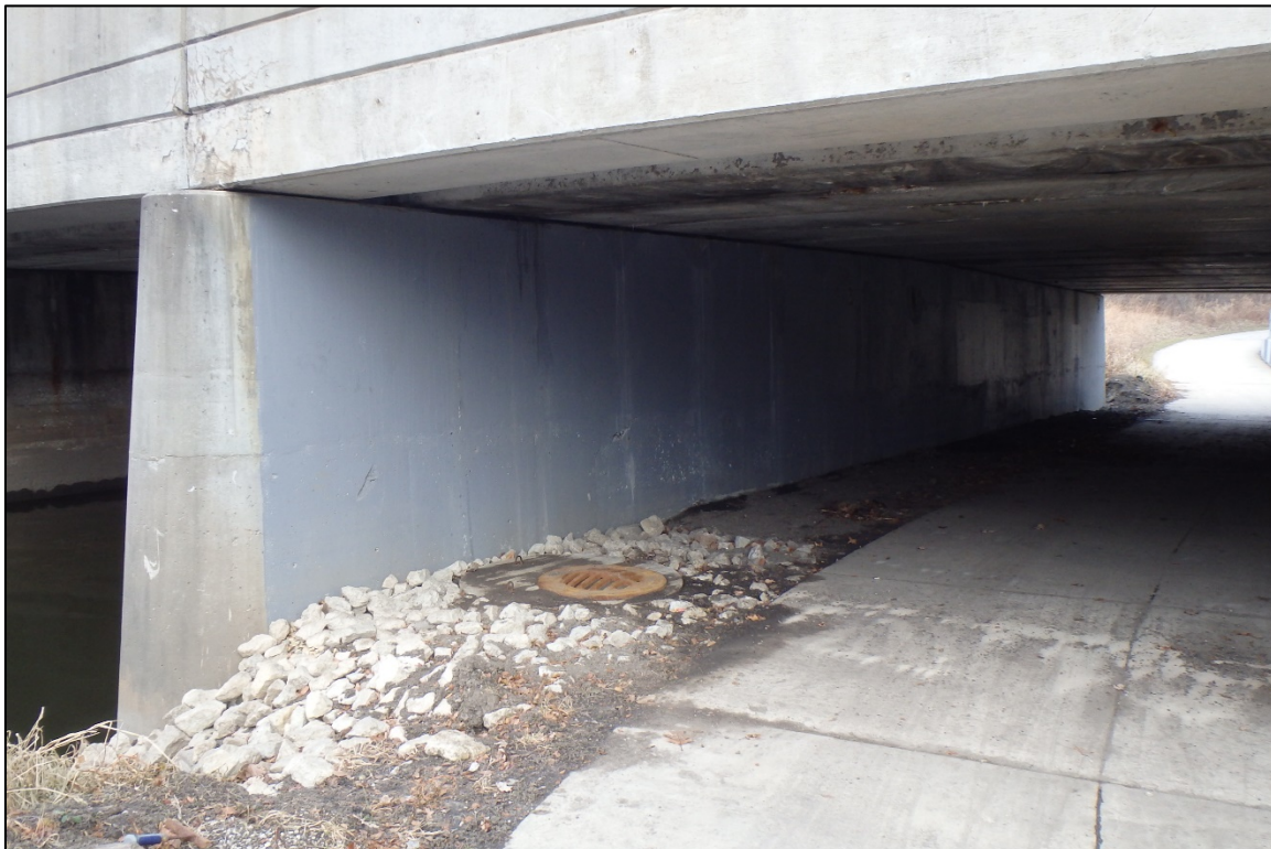
Photograph 16: View of the East Pier, Looking Northwest.
