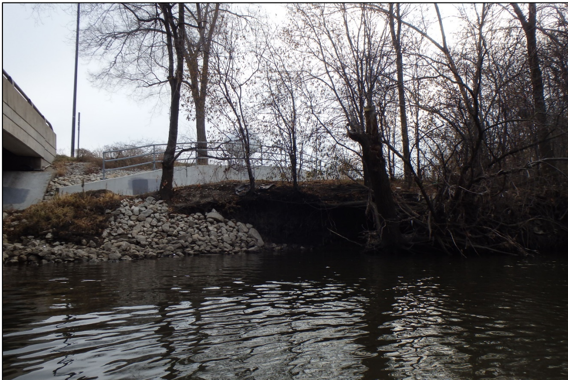
Photograph 6: View of the East Shoreline Downstream of the Bridge, Looking East.
