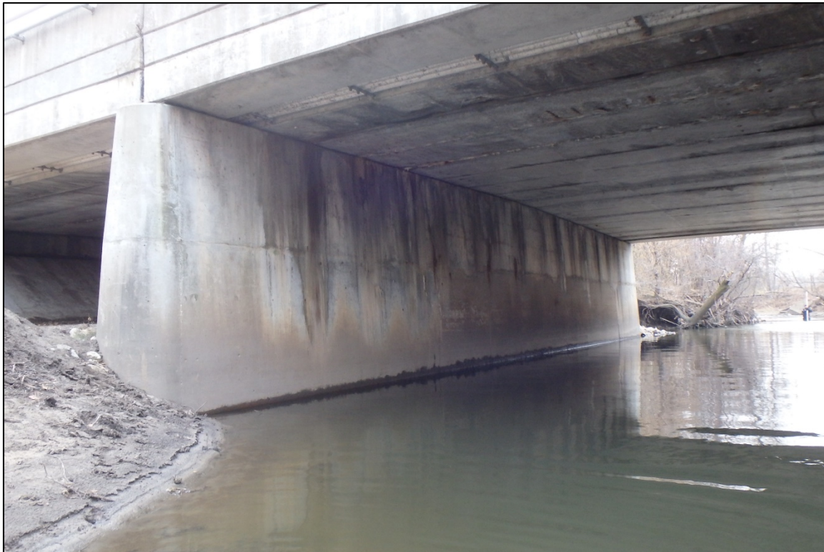
Photograph 17: View of the East Pier, Looking Southeast.
