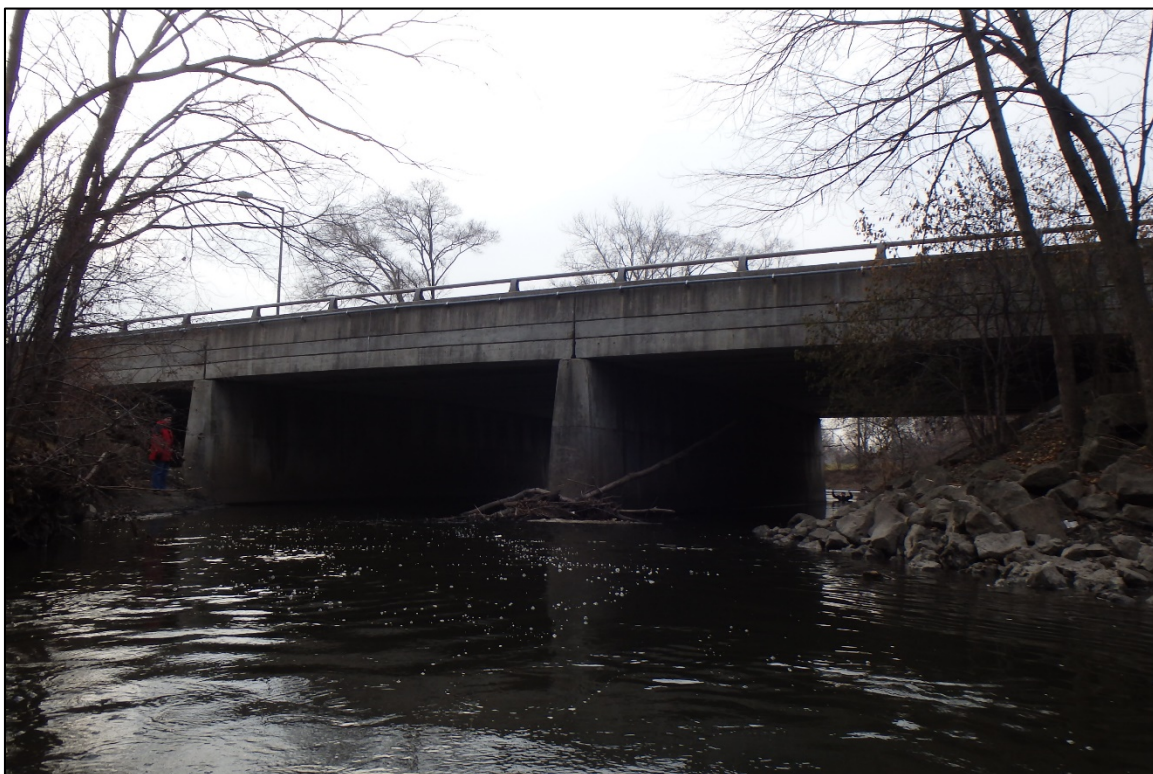
Photograph 2: Overall View of Bridge No. 022-6950, Looking Southeast.
