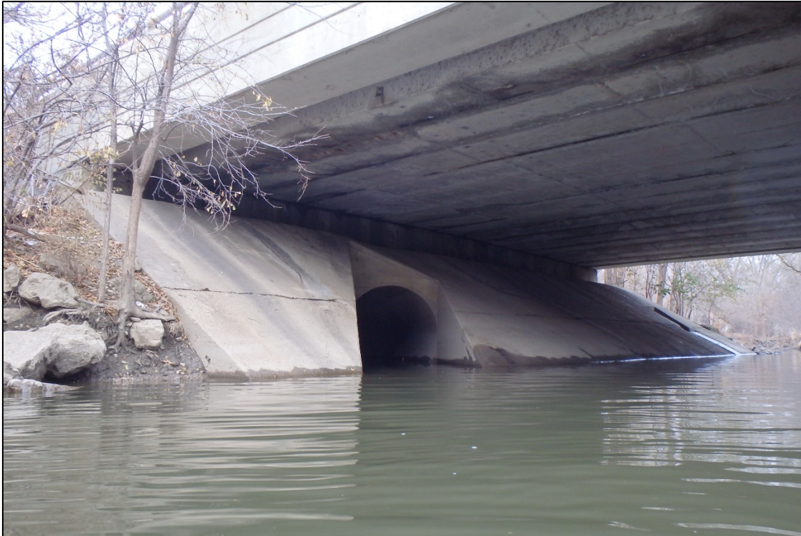
Photograph 7: View of the West Slope Wall and the Abutment, Looking Northwest.
