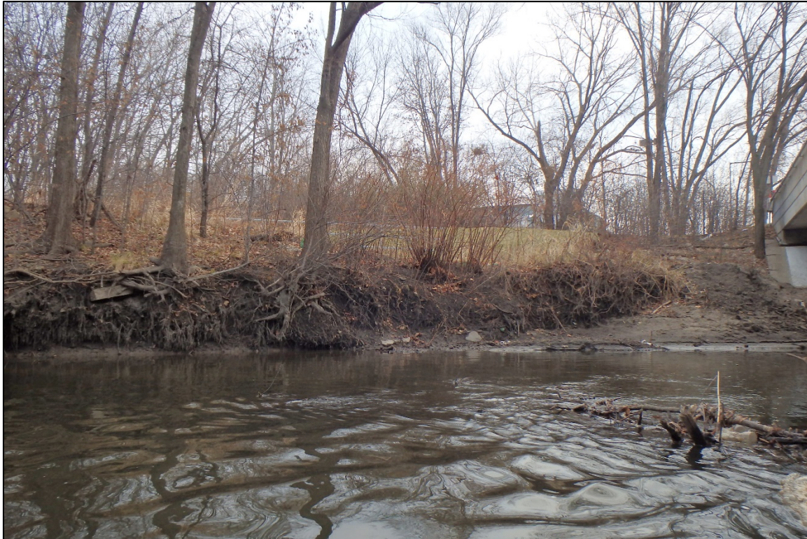
Photograph 5: View of the East Shoreline Upstream of the Bridge, Looking East.
