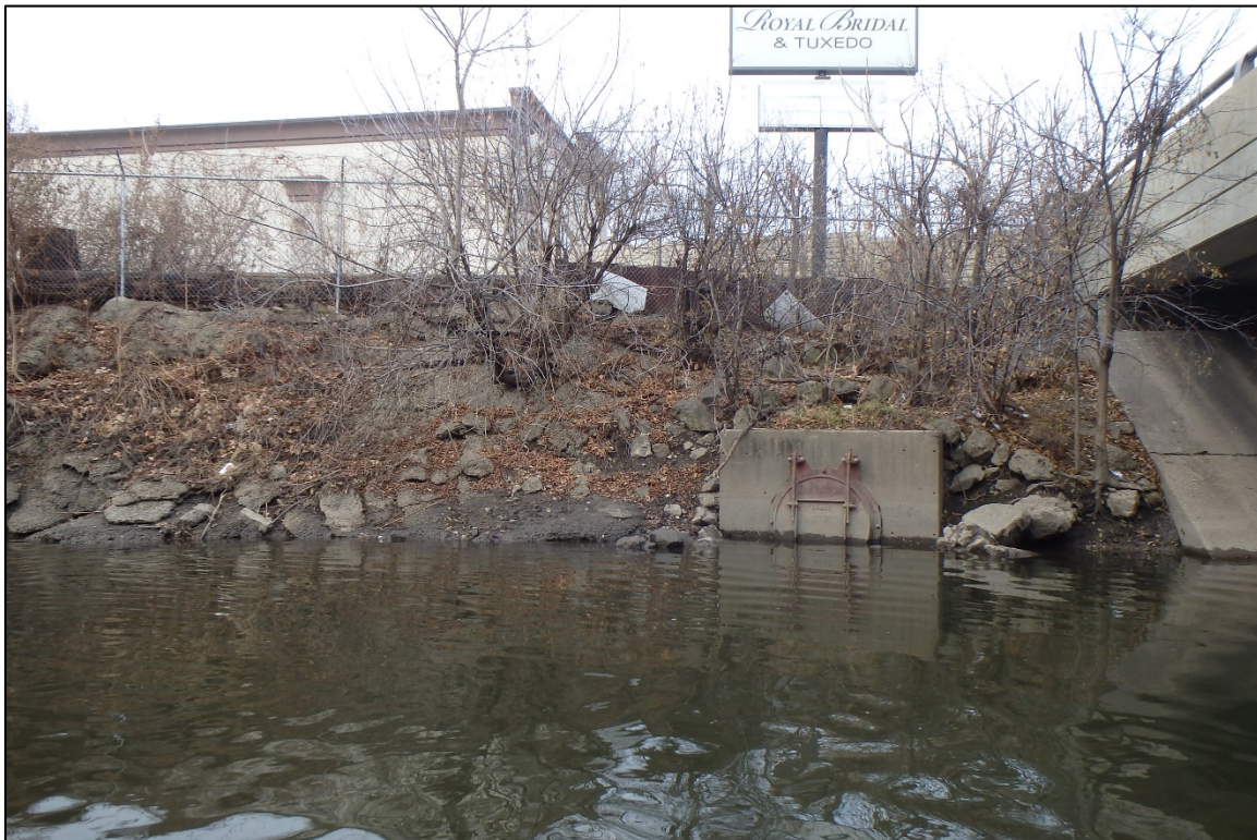
Photograph 4: View of the West Shoreline Downstream of the Bridge, Looking West.
