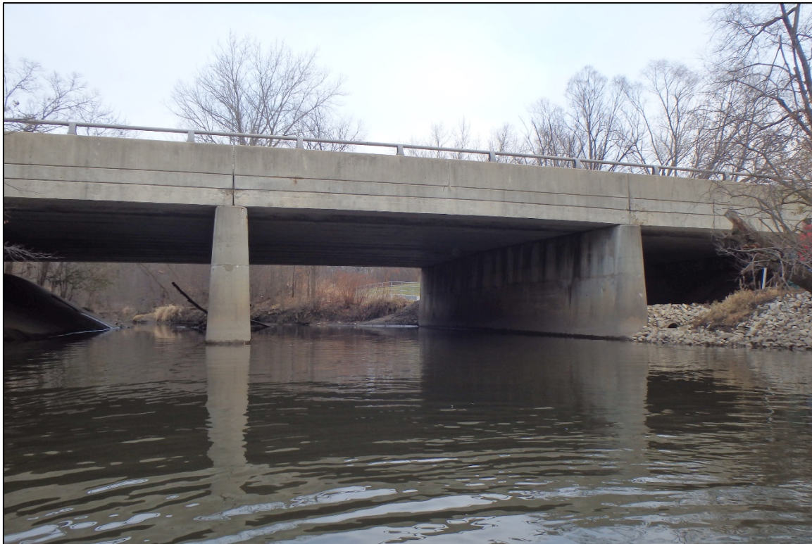
Photograph 1: Overall View of Bridge No. 022-6950, Looking North.
