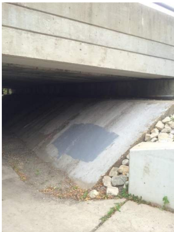
11. Salt Creek Greenway Trail south of St. Charles Bridge (facing northeast).
